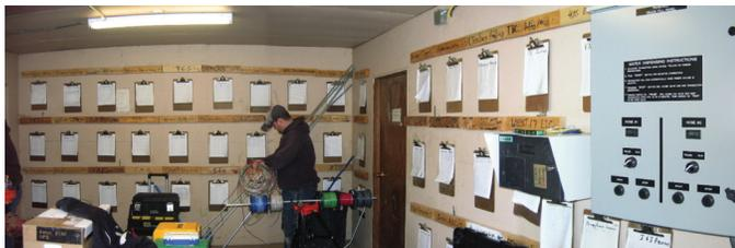
The city of Parshall’s water depot during the installation of their new telemetry system in February 2012. The old billing system of 53 clipboards are still hanging on the walls. The new telemetry system is at the far right of the picture.
