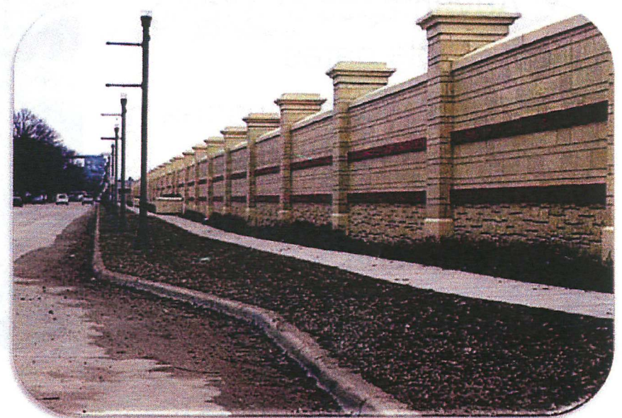
Grand Forks Floodwall
