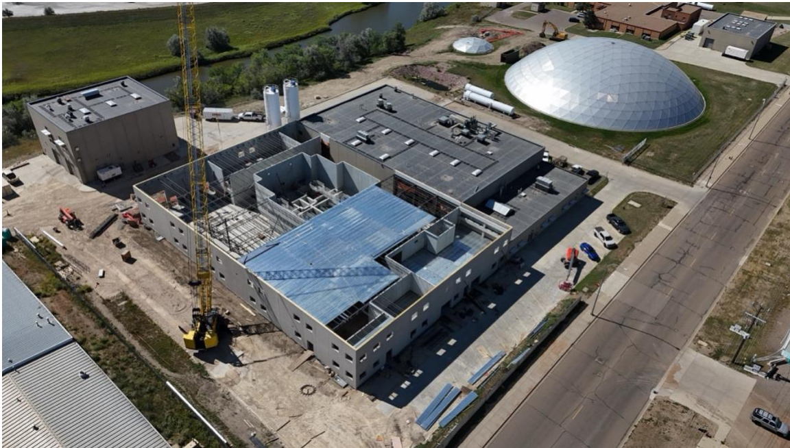
SWTP project picture taken September 9, 2026.
