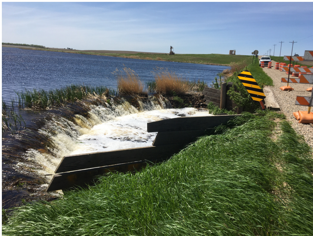
Figure 3. North Star Dam spillway
