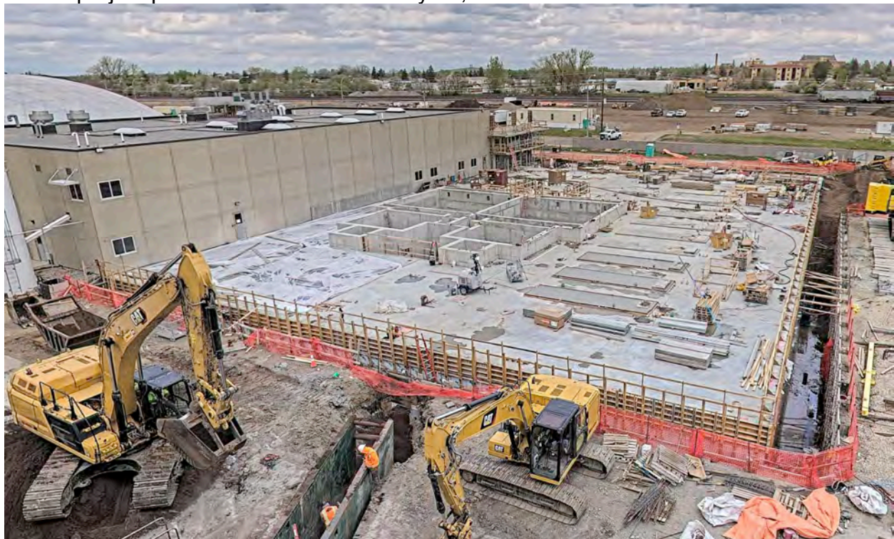
SWTP project picture below taken on May 21, 2026
