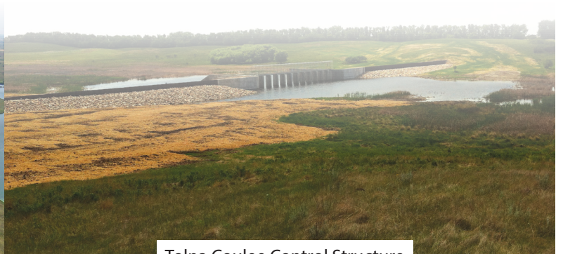
Tolna Coulee Control Structure
