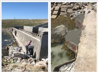
Construction at the Outfall Structure on the Devils Lake East End Outlet features a high-strength, abrasion resistant concrete repair mortar.
