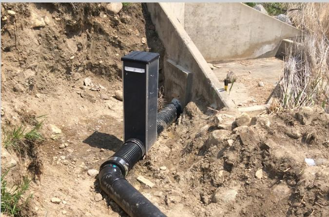
View of the new low-level outlet pipe, entering the principal spillway structure.
