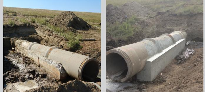
Prior to repairs, the footings for the pipe were deteriorating. After construction was finalized, the pipe was intact and reinforced.
