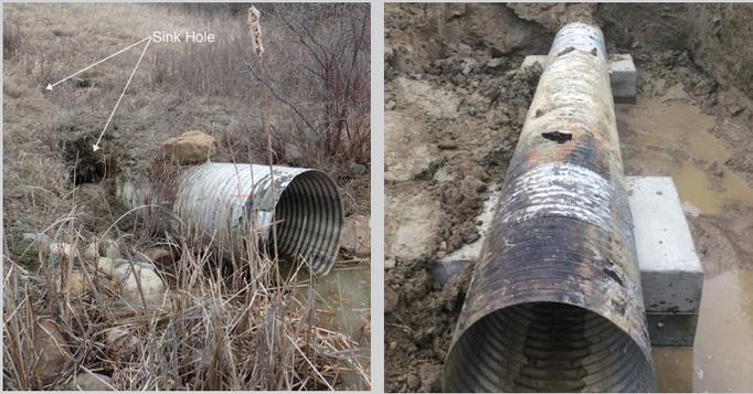
Before repairs were conducted, sagging and warping of the pipe and a sinkhole was forming. The pipe is shown with new supports after repairs were completed.
