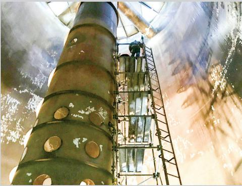
SWC construction crew members cutting additional holes in the center core of a standpipe.
