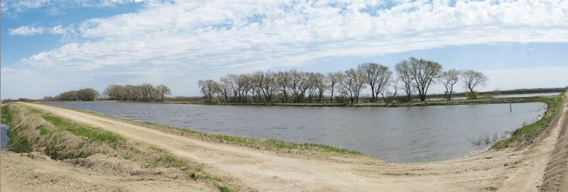
ASR project in Grand Forks County where as much as 1,000 acre-feet per year is added to the Inkster aquifer through an infiltration basin. Water is pumped from the nearby Forest River when flows are high in April to June and later extracted from the aquifer during the irrigation season.
