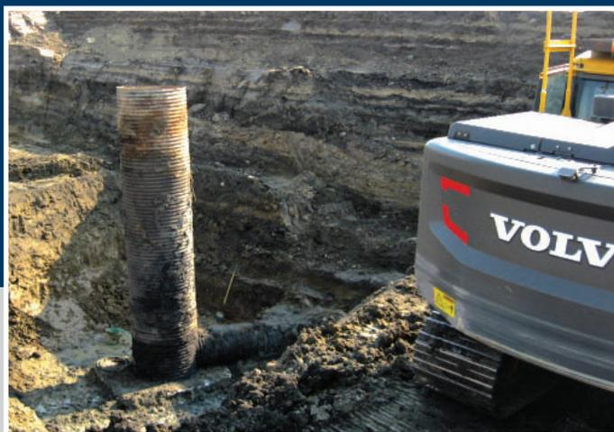
The Construction Crew built a coffer dam around the intake structure to keep their work area dry. The structure was excavated to expose the separated conduit joint, and concrete collar was then constructed around the pipe to seal the joint. The excavation was then backfilled and the coffer dam removed.
