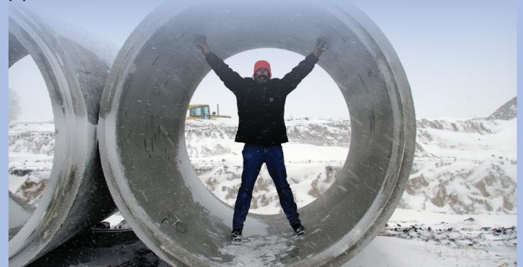
Bruce Engelhardt inside a 96-inch diameter section of a concrete pipe at the construction site of the East Devils Lake Outlet.
