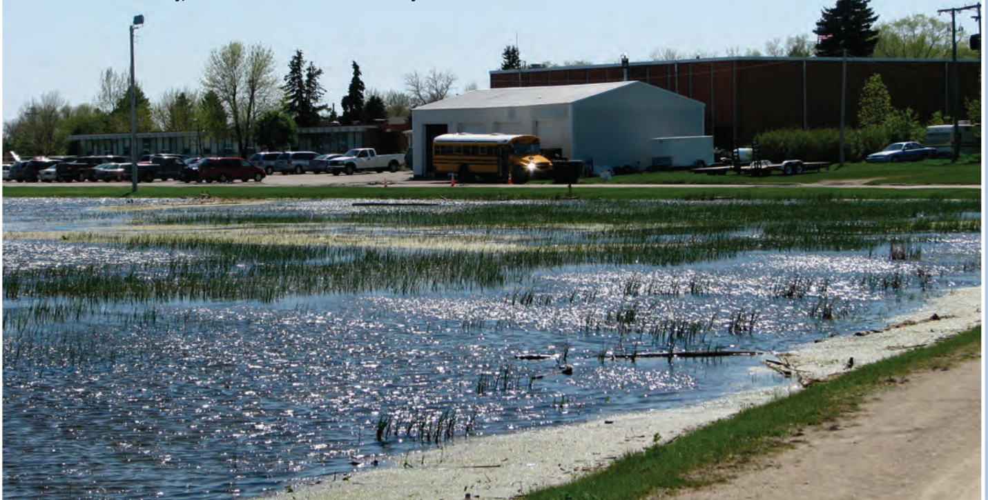
Pictured here is the Minnewaukan Public School, which is only a few feet above the current lake elevation. Some of the recommendations in the new report focus on potential next steps for this small community, which is also the Benson County seat.
