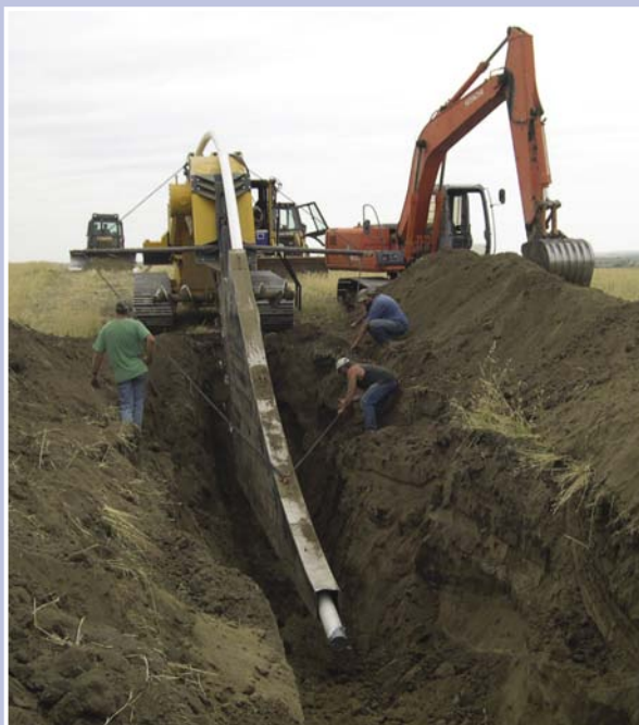
Construction on Southwest Pipeline, Summer 2006.
