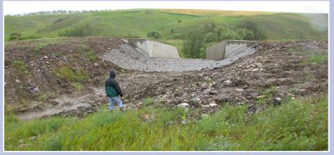
Inspection of reno mattresses filled with rock riprap at Armourdale Dam.
