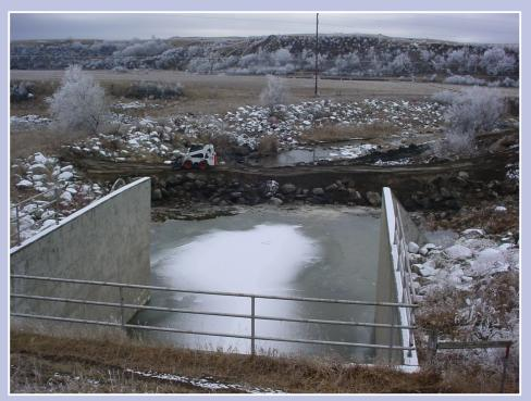
Earth-fill cofferdam downstream of the stilling basin at Sweetbriar Dam.
