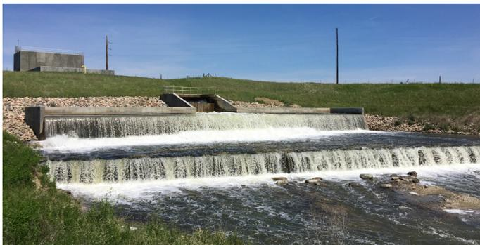
The repairs began in July 2017, with the construction of an earthen coffer dam. This was followed by excavation of the riser and conduit. Forms were then placed around the existing RCP conduit to create a reinforced concrete collar around the separated joint. The structure was then back-filled and the cofferdam was removed. The borrow site was reclaimed and seeded.
