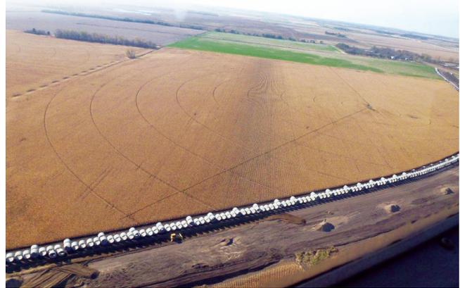
be located in the Tolna Coulee above the Town of Tolna. The project includes 5.5 miles of 96-inch pipe, five pumps at the intake structure, and a rock filter and stilling basin at the outfall structure. Completion is scheduled for June 2012.
