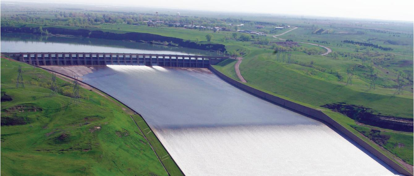
On the morning of June 1, 2011, 7 of 28 spillway gates were opened at Garrison Dam for the first time ever to release floodwater.
