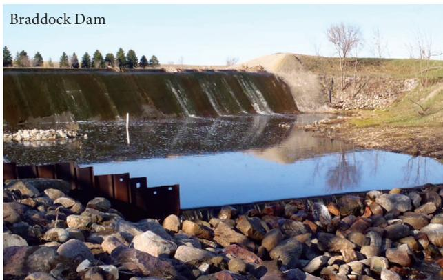
caused the leftmost 20 feet of the sheet piling to collapse. The erosion removed an estimated 600 cubic yards of material, including the rip-rap along the downstream face of the weir. It appears that the flow may have completely overtopped the stilling basin weir, starting the erosion around the ends of the weir. The scour removed the supporting soils from in front of the 6-foot lengths at the wings, causing the left side to fail by overturning.
