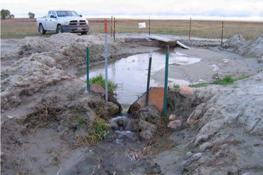
*SWC's Appropriation Division constructs a weir to measure the rate of water discharge from a flowing drill hole.*
