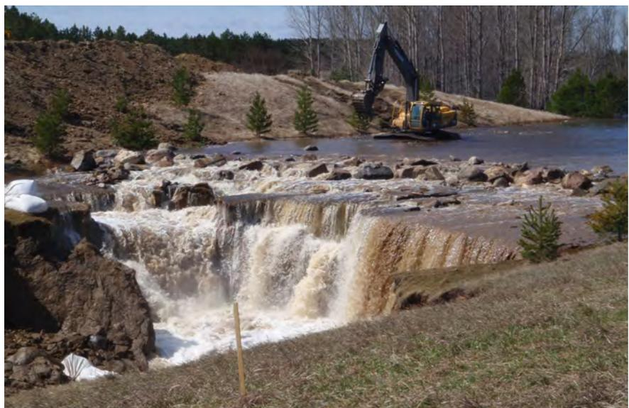
*SWC Construction Crew used a track hoe to slow erosion of the spillway at Cottonwood Creek Dam by placing rip-rap.*
