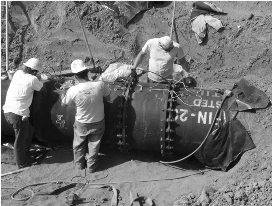
*Workers are placing cathodic protection on the pipe for the Northwest Area Water Supply project south of Minot.*
