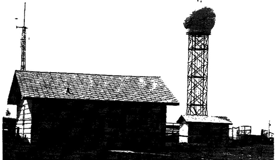
*The Bowman radar, sited at the Bowman County Airport. The transmitter and receiver are housed in the building at the base of the tower (right), and the console and operations computers within the office building (left). Both buildings are provided by the Bowman County Airport Authority. (Photograph by Bruce Boe)*
