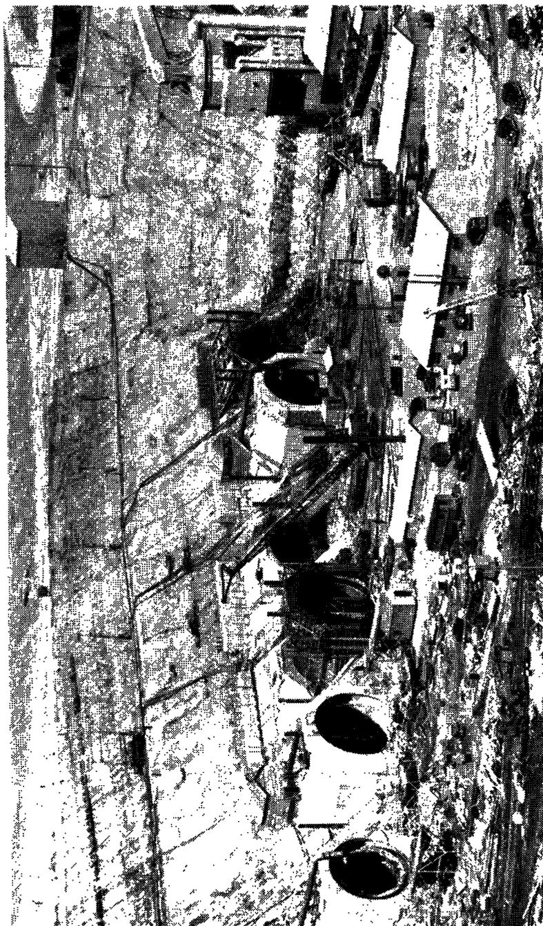
Garrison Dam Tunnel Outlets in Process of Completion — Cement Mixer at Right
