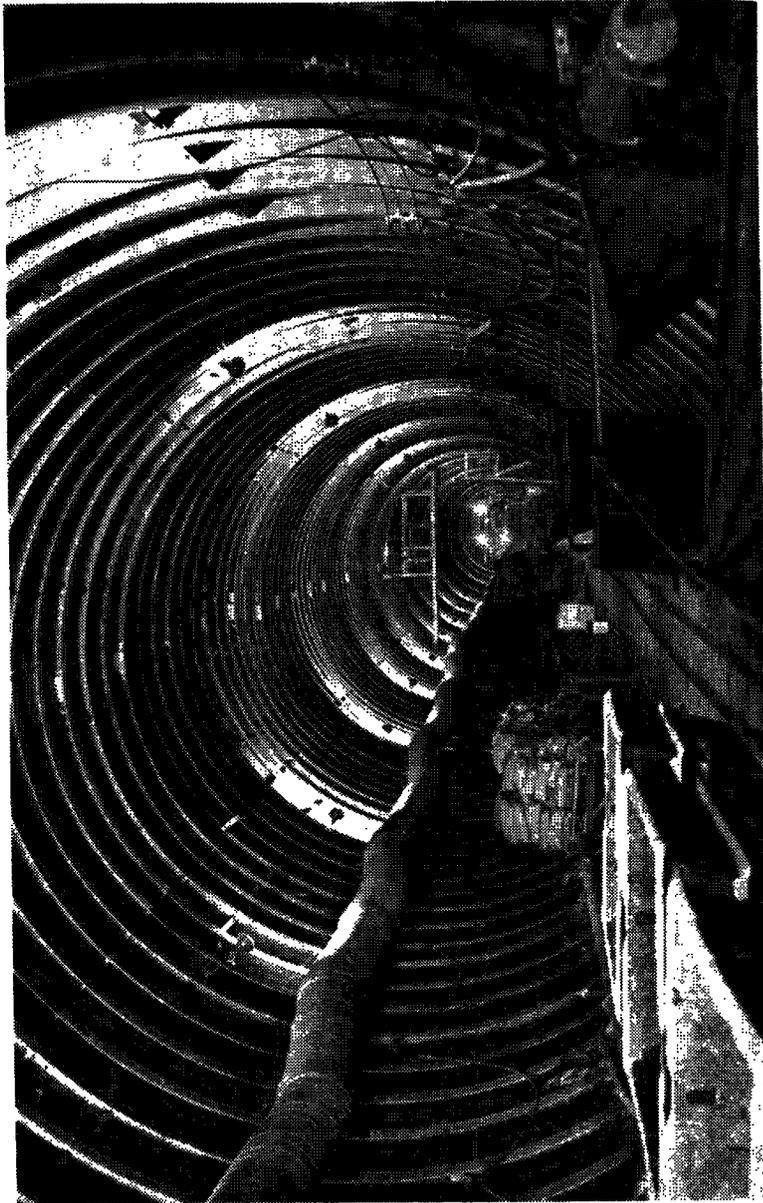
Garrison Dam 36 ft. Diameter Tunnel in Process of Construction
