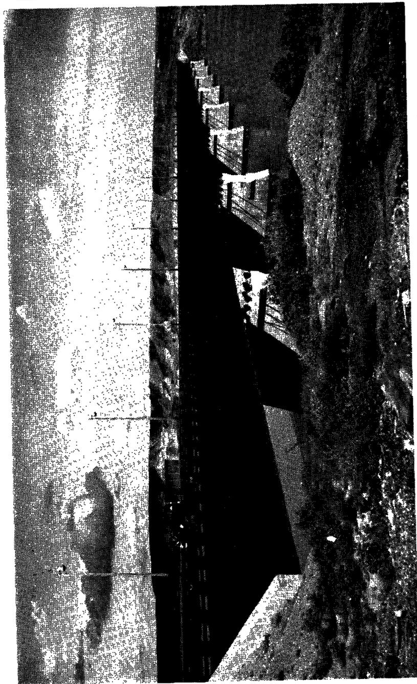
Garrison dam bridge was built for construction purposes. It carries both railroad, truck and passenger cars for hauling materials and construction workers.
