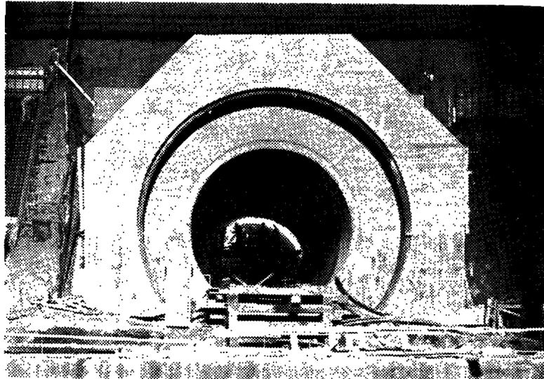
Floodlights enabled the photographer to take this night picture of the upstream portal of tunnel No. 7, recently completed. This tunnel is 22 ft. in diameter and required 10,947 cubic yards of concrete in the 3½ ft. thick lining.
