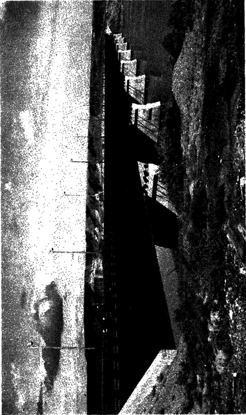
Garrison Dam Construction Bridge carries foot passengers, trucks and trains, and from which Trainloads of rock will be dumped to close river channel
