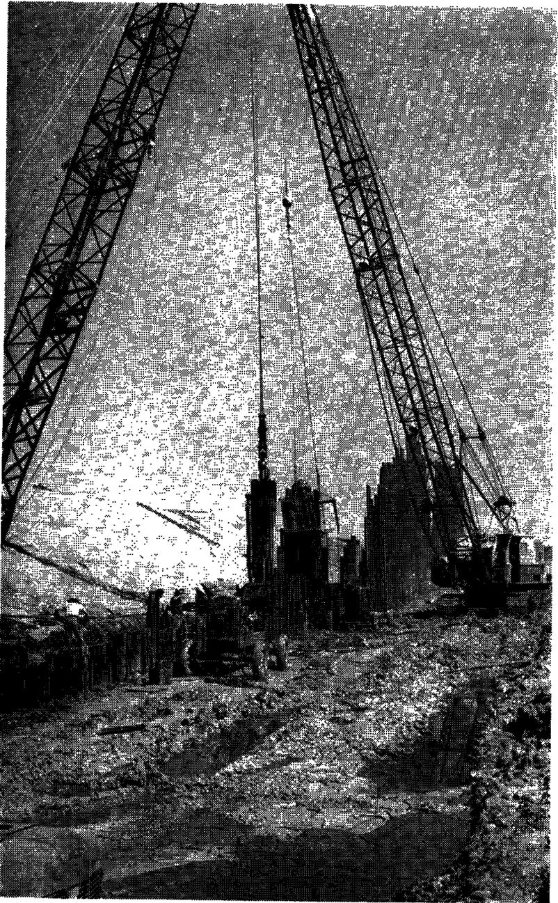
Driving Steel Piling Cut-off at Garrison Dam
