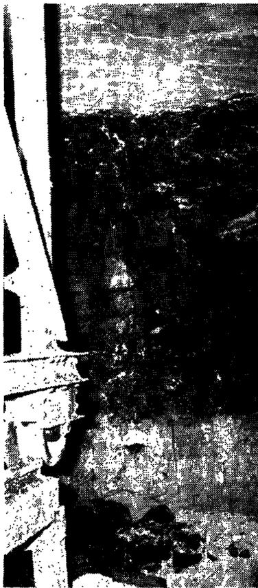
Lignite eight feet thick has to be cut through in the tunnel. The lignite separates two strata of clay, at the Garrison dam.
