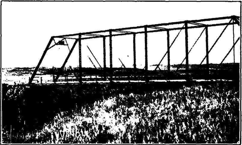
Old Bridge Over the Knife River in Mercer County. An Example of a Bridge Designed for a Very Light Load. Note the Poor Foundations.
