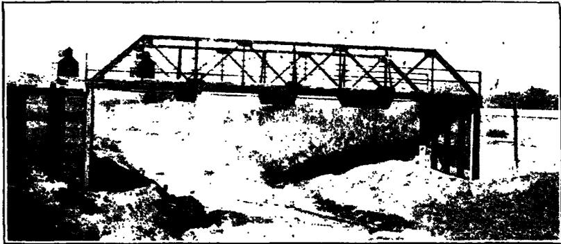
Mercer County Bridge. An Example of a Very Good Steel Truss Placed On a Poor Type of Abutment.
