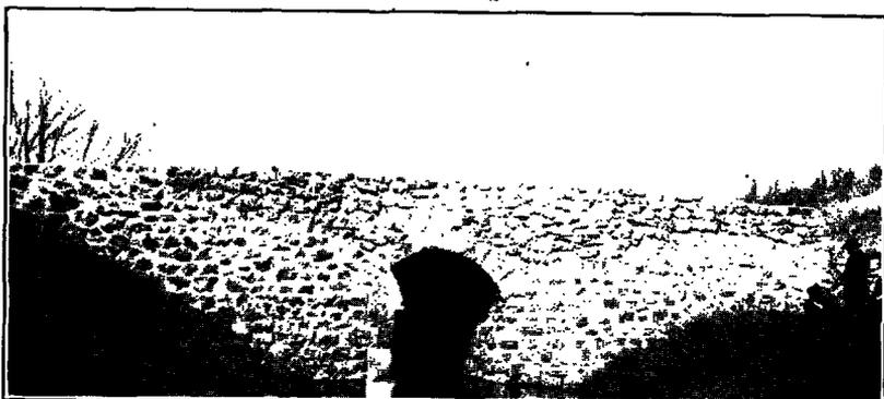
Masonry Arch on Square Butte Creek, Oliver County. Span of Arch is 10 Feet and is Too Small. Cost of Work at This Point \$1,500.
