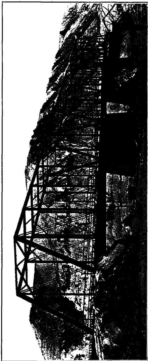
Bridge Over the Little Missouri River at Medora. Designed by the State Engineer's Office. Built by the Illinois Steel Bridge Company of Minneapolis. Length 405 Feet. Total Cost of Bridge and Approaches, \$20,000. Courtesy of Doubleday & Myers, Dickinson, N. D.
