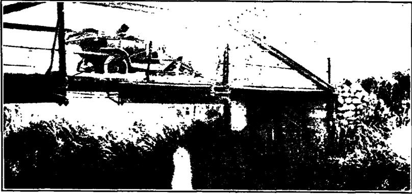
Bridge in Mercer County. Note Damage Done by Ice, and the Poor Type of Abutment.
