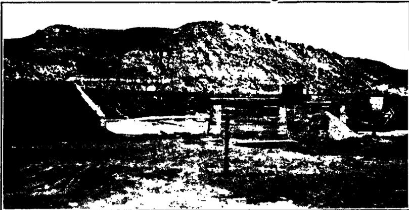
Medora Bridge, Showing One Abutment and Two Piers Complete, Work Being Done on West Abutment. Work Being Done in December. Water, Sand and Gravel Being Heated and Forms Protected For Ten Days
