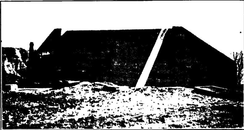
Medora Bridge. Gravity Type Concrete Abutment. 15 Foot 12 Inch Piling Driven to Refusal at Three Foot Centers Were Driven in Bottom of Excavation. The Man is Standing on Top of a Two Foot Concrete Footing
