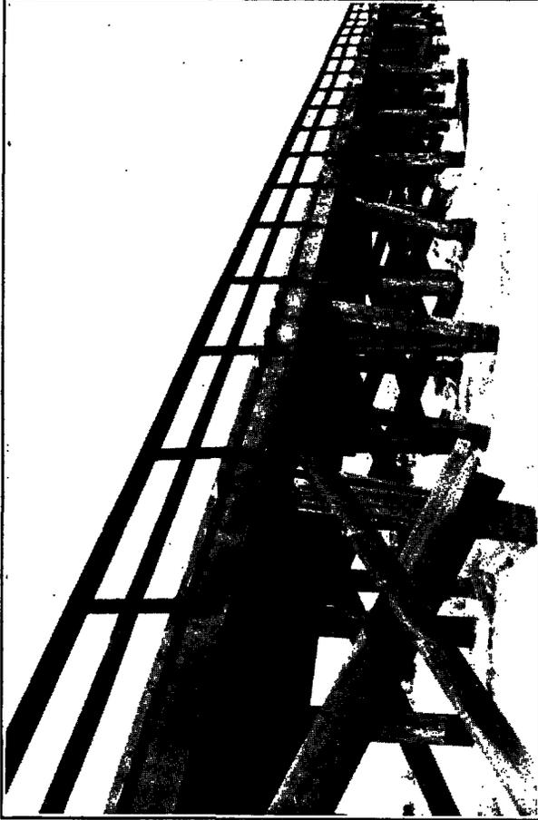
A Wooden Pile Trestle Over the Des Lacs Lake. Note How the Weaker Ice Under the Bridge Buckled on Account of the Pressure Exerted by the Expanding Bodies of Ice on Either Side. Piles are Broken Toward the Center of the Bridge.
