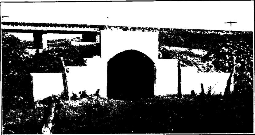
Reinforced Concrete Culvert and Cattle Pass Near Baldwin,
